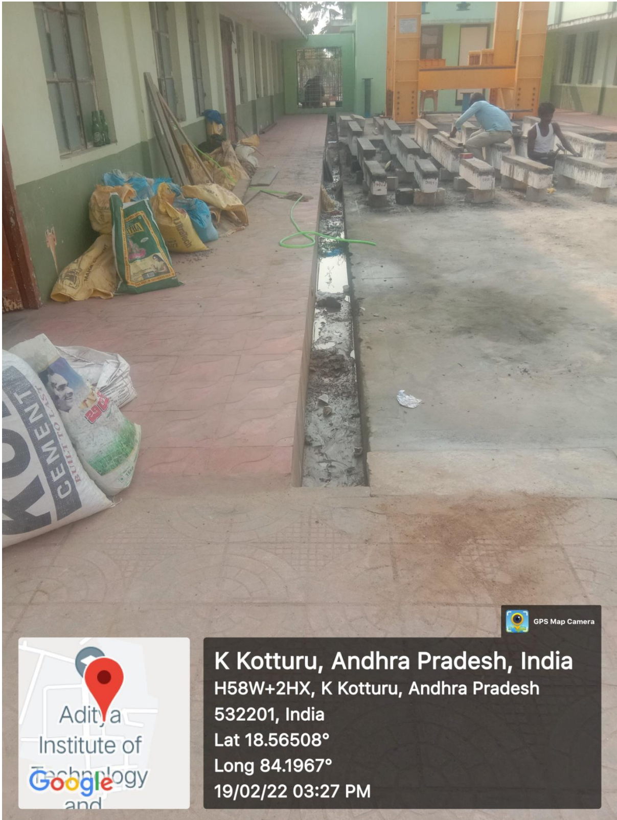
Sub drain for storm water collection
